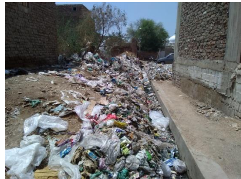
Figure 8:9: Drain full of Solid Waste
