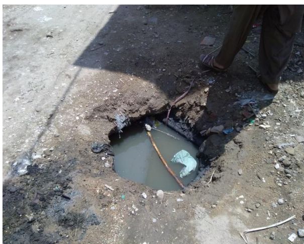
Figure 8:5: Broken Drains
