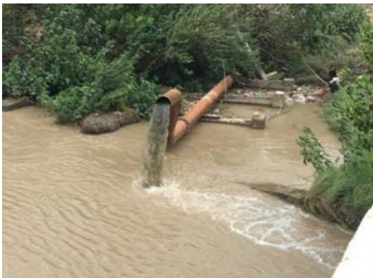
Figure 8-6: Raw Sewage Discharge from Pumping Station
