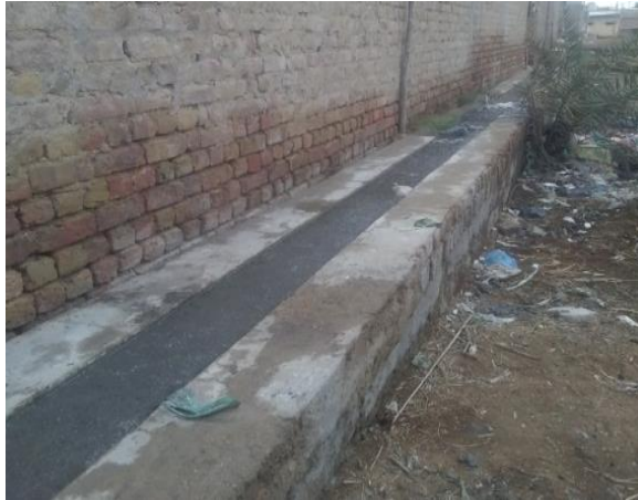
Figure 8-4: Non Functional Drain
