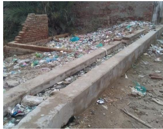
Figure 8-5: Non-functional Drain
