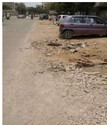
Figure 2.18: Picture of ill maintained buried sewerage line at Strachan road with open manhole
