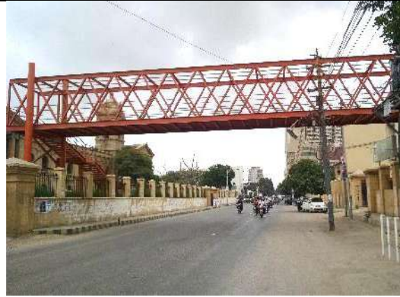
DJ Science College Pedestrian Bridge connecting old and new buildings across the road. The entry and exist of the bridge is located inside the buildings. No connection from the road.
