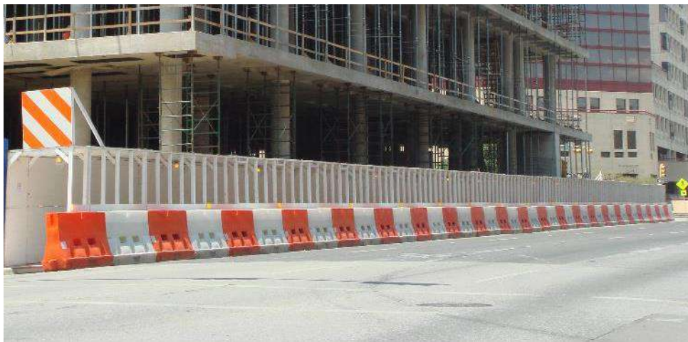
Figure 6.2: Hard barricade for construction site along the road with access to pedestrian
