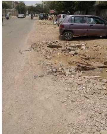
Figure 5.5: Picture of ill maintained newly buried sewerage line at Strachan road with open manhole
